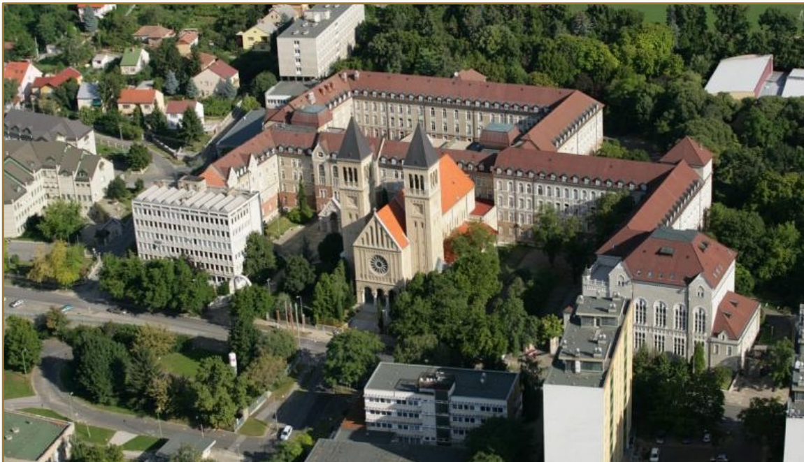
A faculty building of the University of Pécs.
